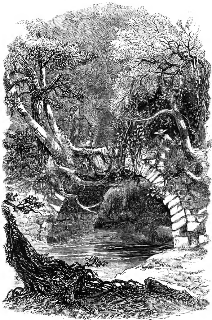
ANCIENT BRIDGE AT OLD PANAMA.
